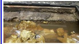
Our burst pipes have caused water to fill the underfloor pipework ducts this is beside the main entrance.
